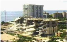
This is a picture of a controlled demolition of a building. The white puffs of what appear to be "smoke" are actually explosive debris generated by explosive shaped charges cutting the main structure of the building. These blown in sequence removes these critical supports in such an order to cause the building to fall in on itself.
